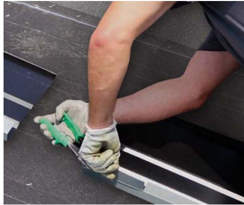
Cut out top leg of inner gable trim to allow for tight, waterproof overlapping.
