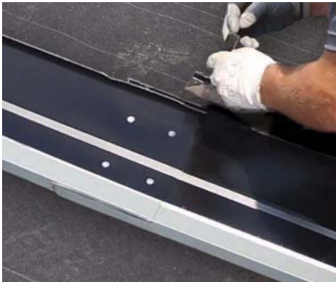
Install inner gable as a whole piece. When adding a second inner gable trim, open up the water lock and cut out the top section to allow for tight, overlapping, waterproof fit.
