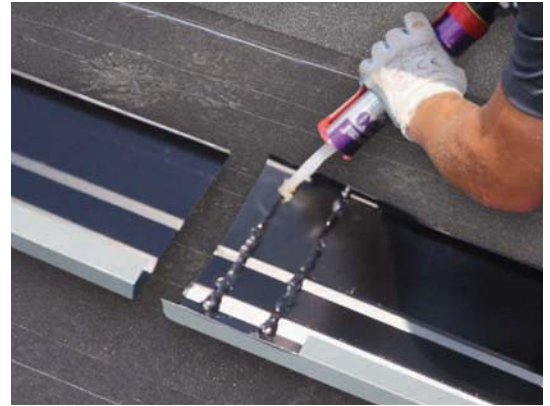
When overlapping, apply sealant under overlap. Be sure to screw every 12" between the diverter and the water lock.
