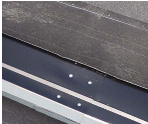
Refit the overlapping water locks together with a hand seamer.
